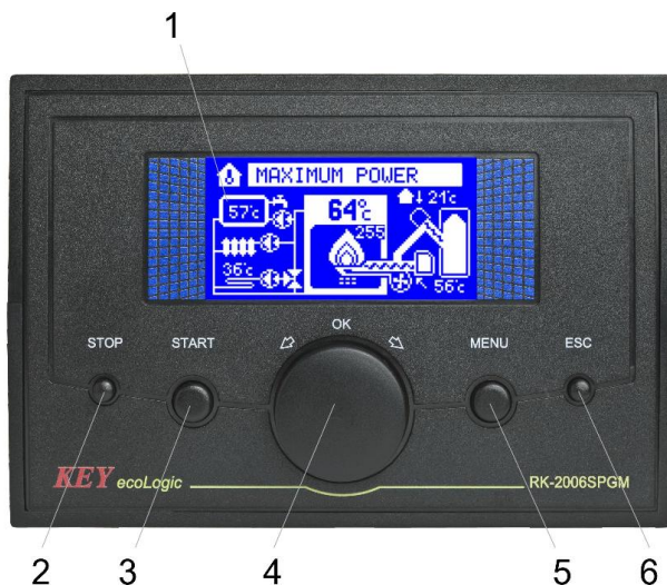
Figure 1. Front panel of RK-2006SPGM controller.
